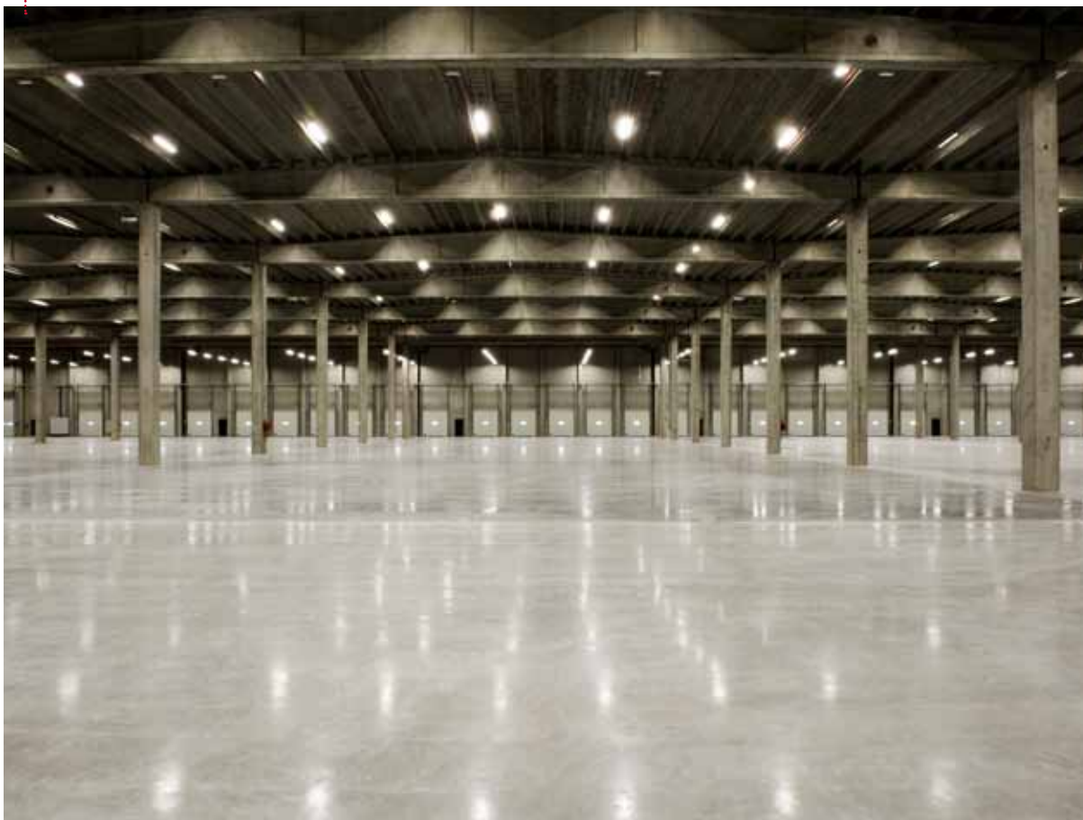
Canal Logistics, Anderlecht © Koen Keppens
