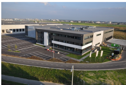
Montea "Space for Growth" – Site Brucargo 831
