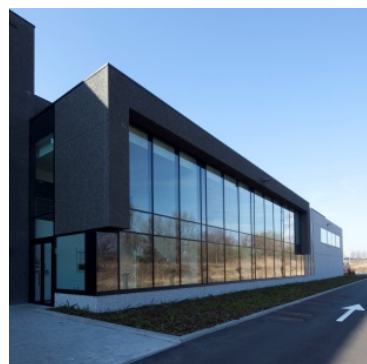
Montea "Space for Growth" – Site Haven Gent Hulsdonk
