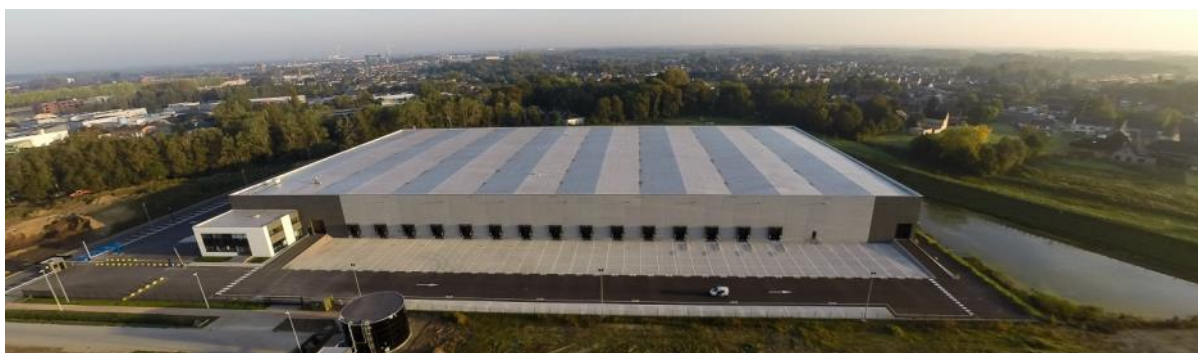
Montea «Space for Growth» - site MG Park De Hulst – Neovia Logistics Services Belgium (BE)
