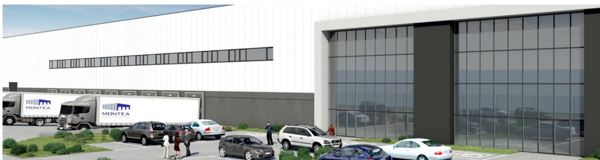
Montea «Space for Growth» - Site Bornem – Build-to-suit (BE)
